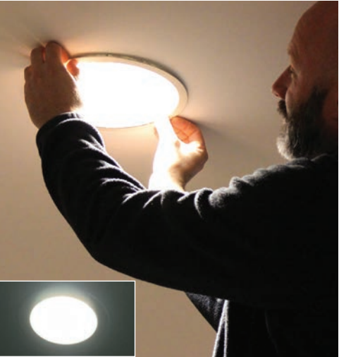
The Foundation underwrote the installation of new LED lighting for better energy efficiency and visibility.
