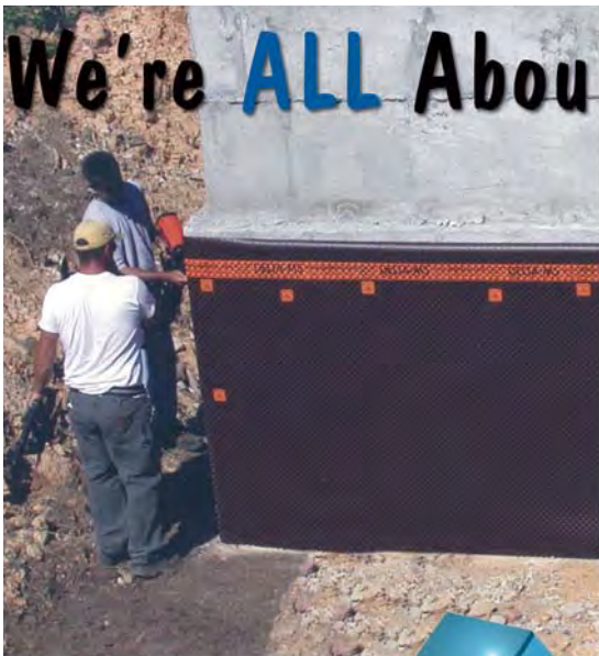
Foundation Drainage
