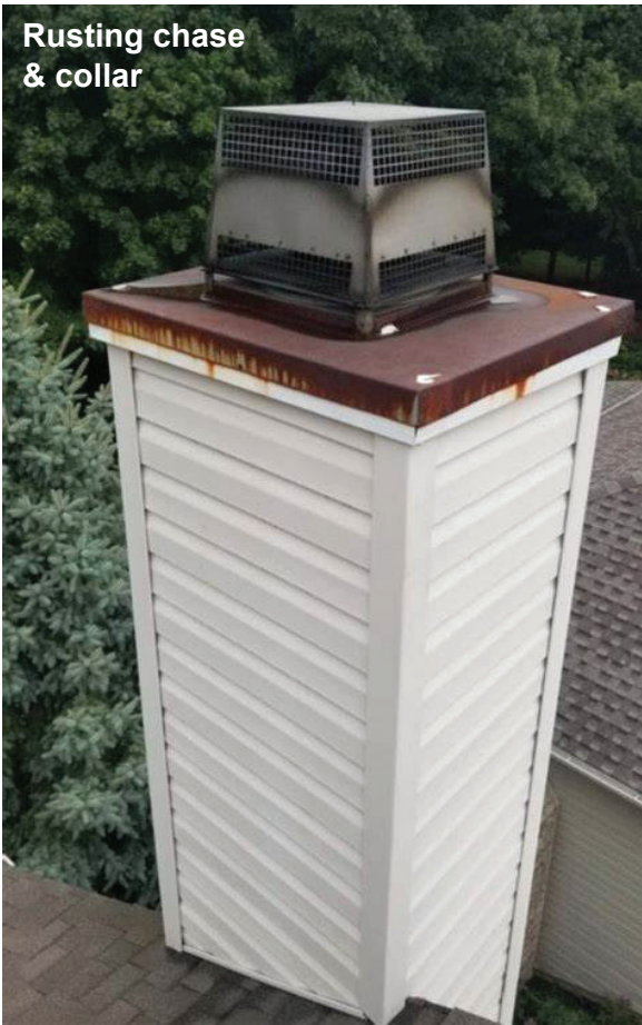
Chimney discoloration due to rust
